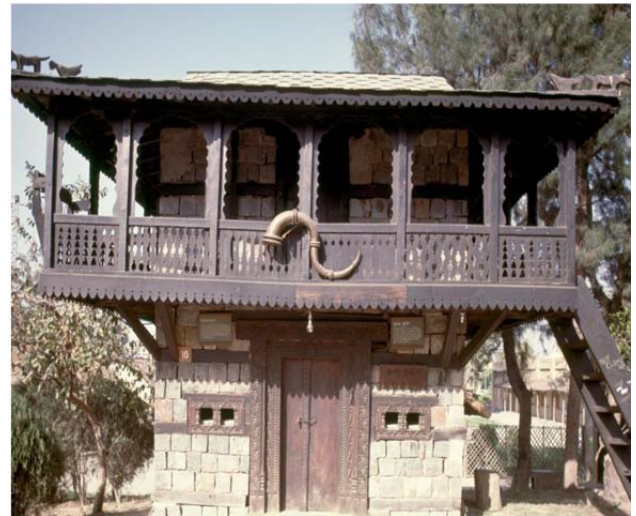
Fig. 8: Structure reflecting the vernacular influence
